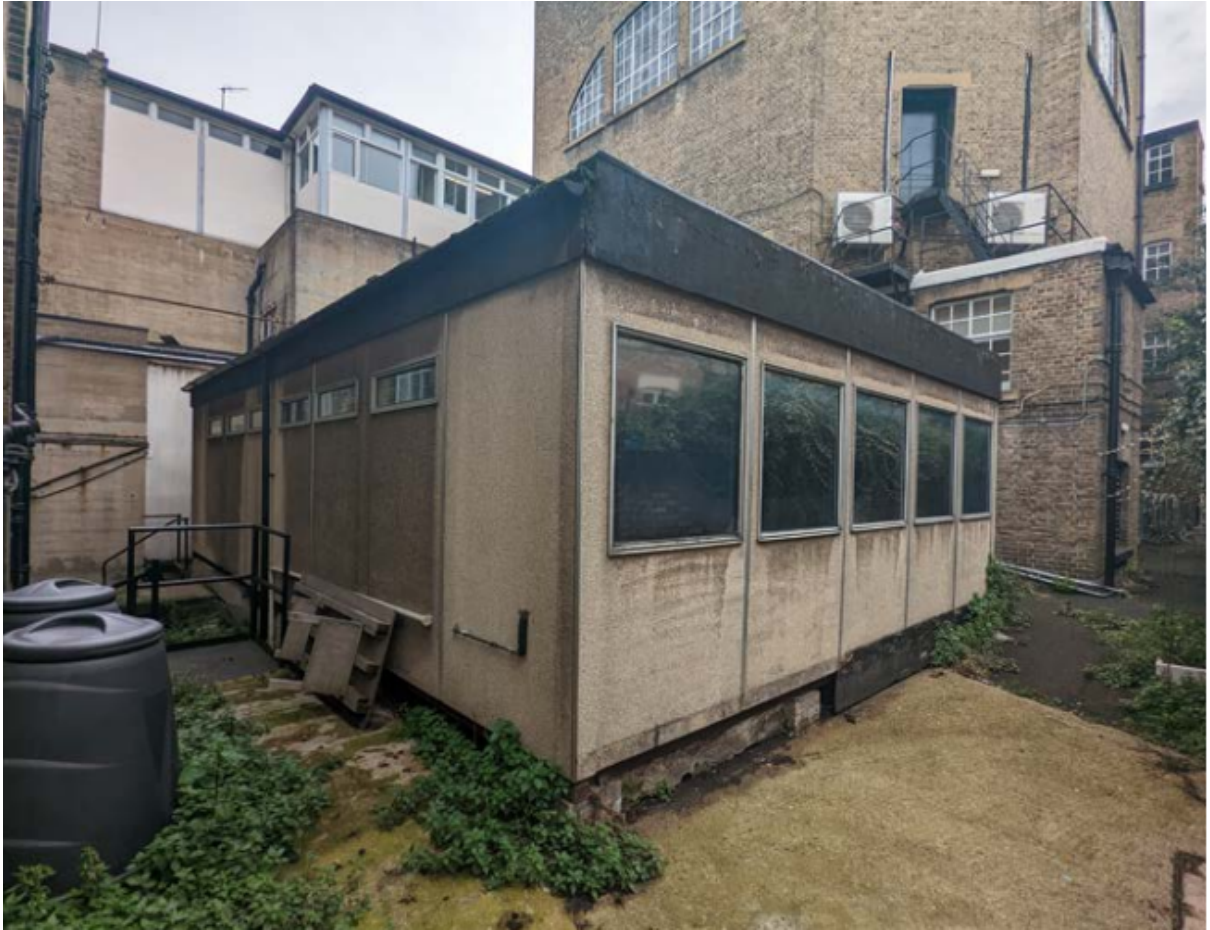
Image 7: Portacabin and paving area
